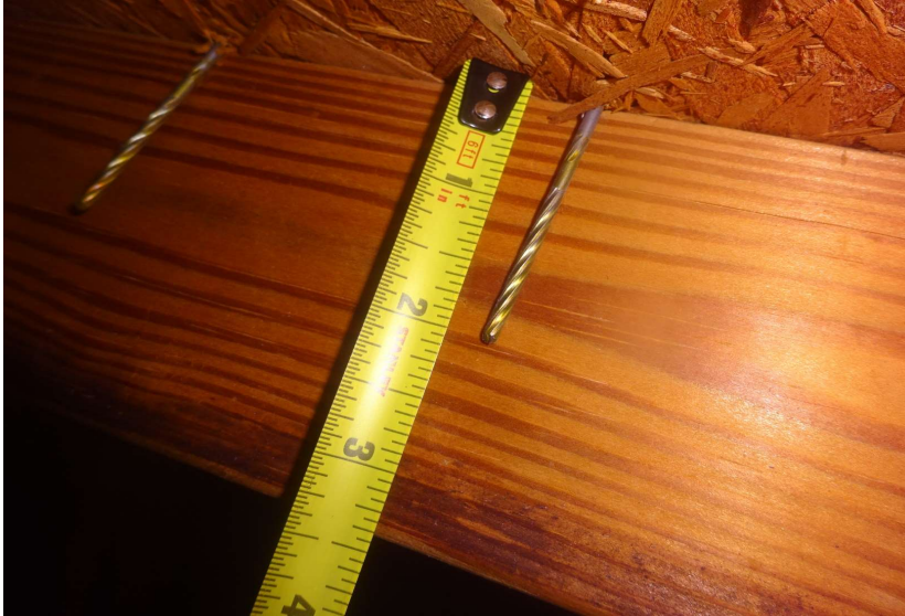
8d nails verified
