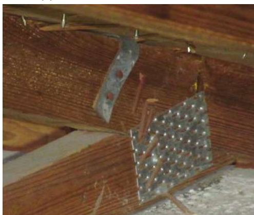
Single wrap with at least 2 nails on the embedded side and at least 1 nail on The wrapped side
