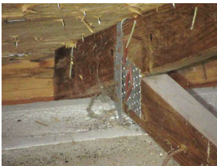
Single wrap with at least 2 nails on the embedded side and at least 1 nail on The wrapped side
