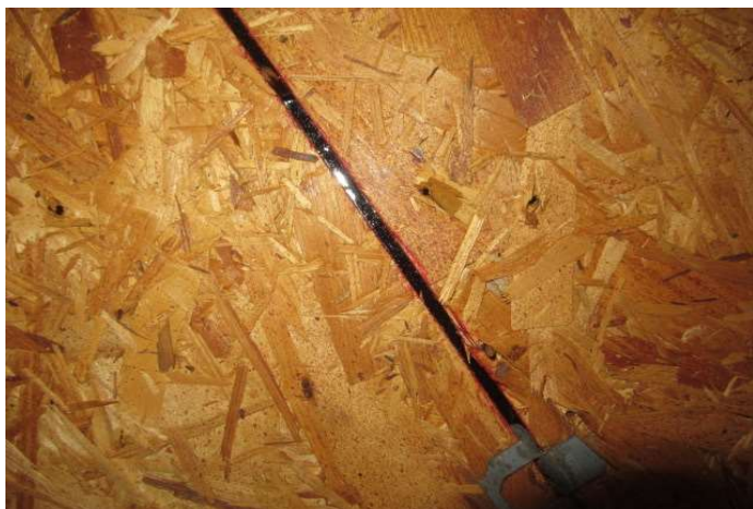
SWR installed under the shingles
