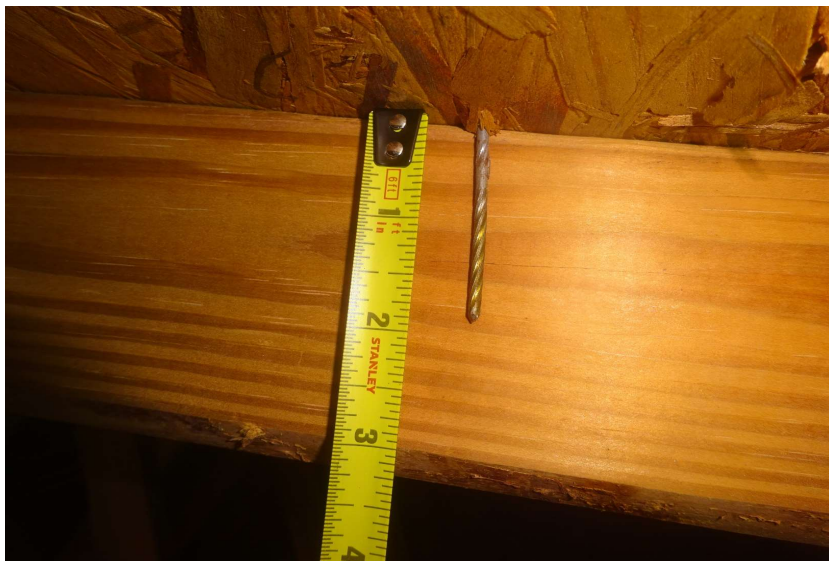
8d nails verified
